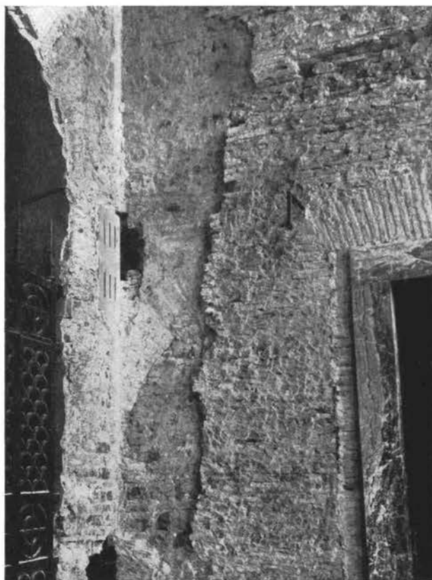
Fig. 17 — S. Lorenzo f.l.m. West basilica, east end of south aisle (intermediate bays), detail, 1947-49 (Photo: Sansaini).
